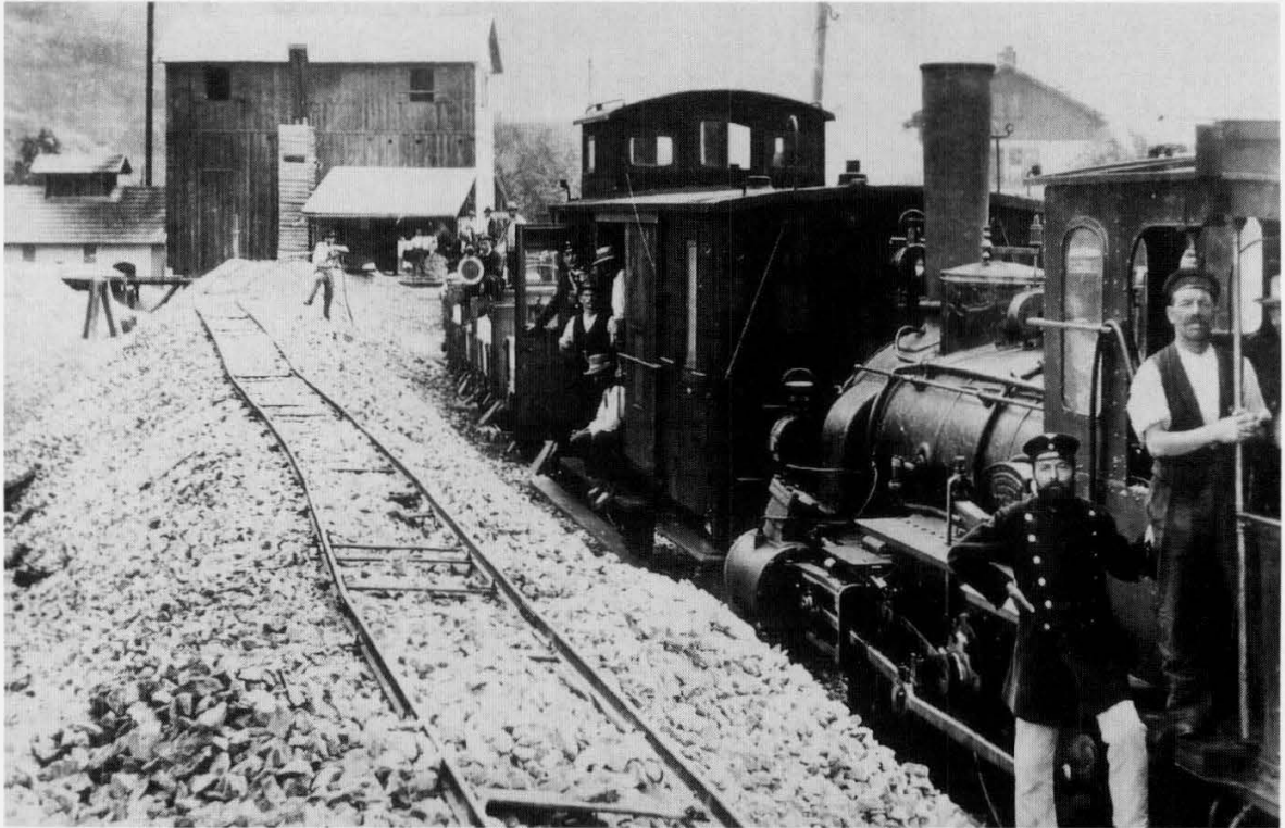
Porphyrverladestation in Hubacker
