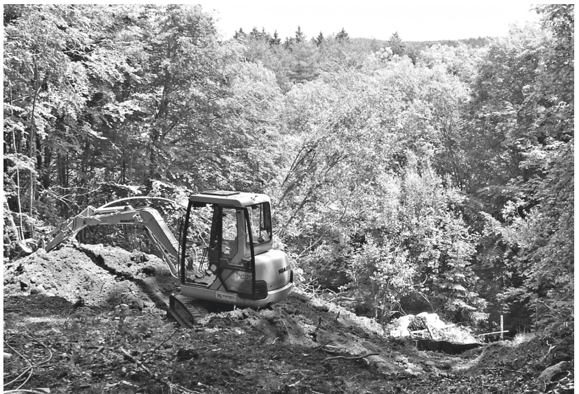
Figure 1. 2005 excavation showing machinery used in preparation of the Western Quarry. – Photographs: by the authors, if not noted differently.
