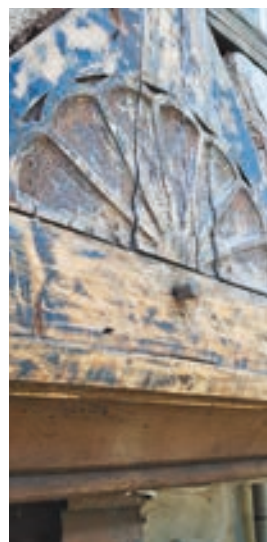
Abb. 4: Obere Straße 37 Erkerdetail, Stadt VS.
