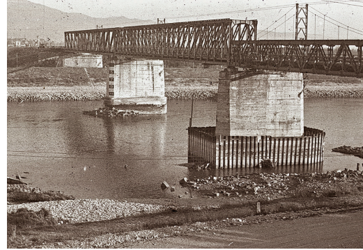
Chalampé–Neuenburg, Notbrücke, 1946 (BAW, HBdia1012)
