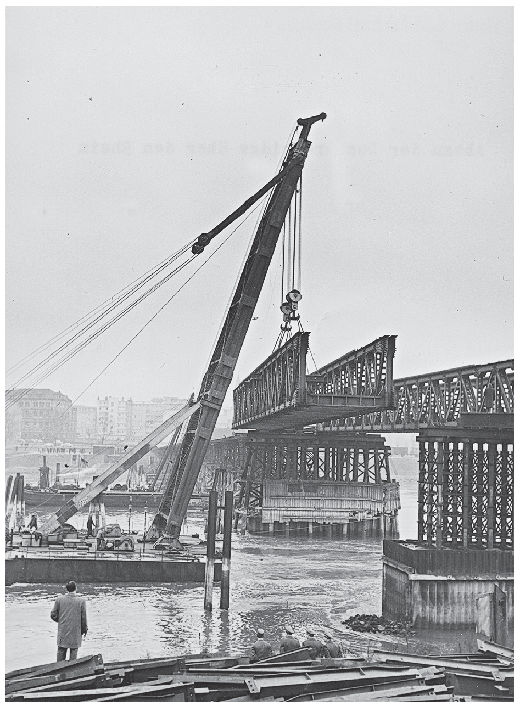
Ludwigshafen–Mannheim, SKR-Brücken, 1948 (BAW, HB12176)
